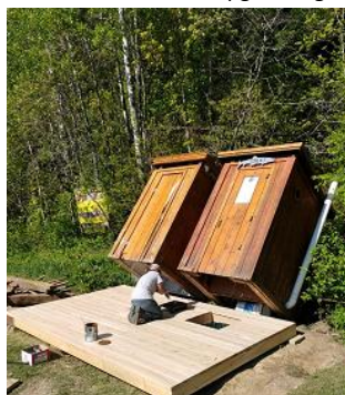
Réfection du plancher au Rafting Ground – Floor renovation at Rafting Ground
